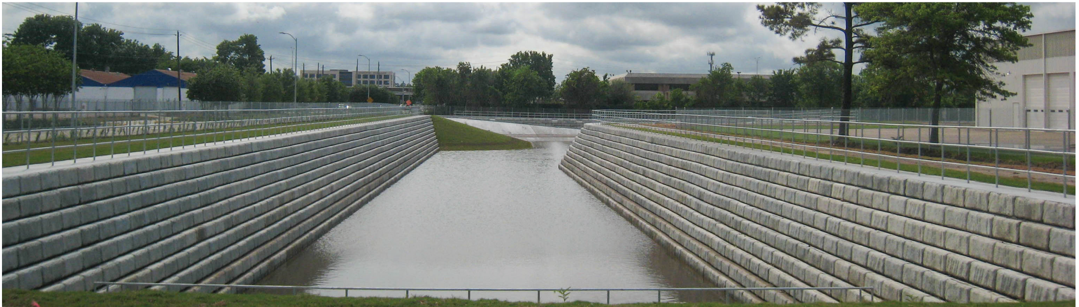
LUMPKIN ROAD DETENTION POND HOUSTON, TEXAS | WILBERT VAULTS OF HOUSTON
